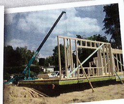
Timber Frame Work
